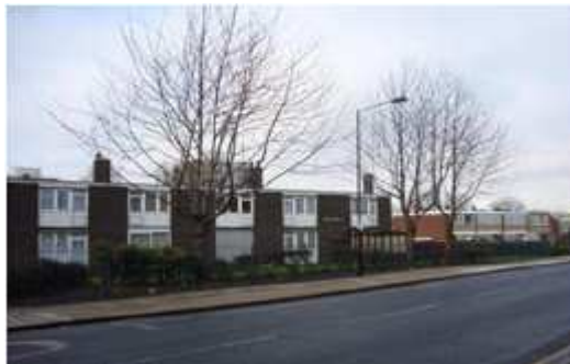
Fig 1: View of previous units (now demolished) on Chrisp Street
